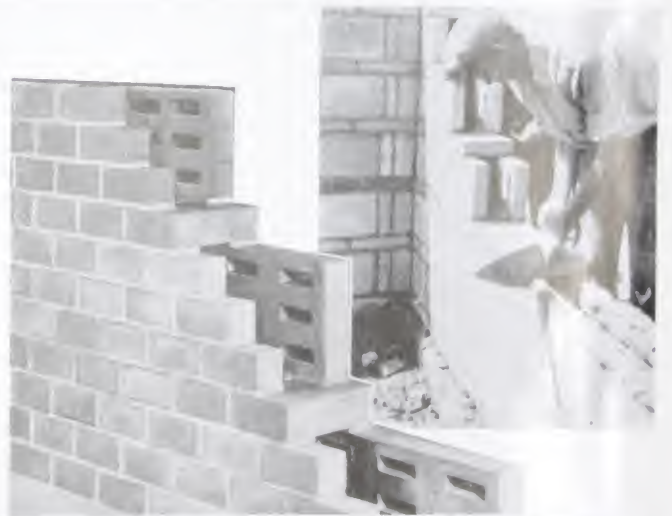
Dunbrik is used in solid and hollow wall construction, plain or faced.
